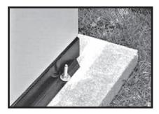
Some locations require the use of a poured concrete mounting pad. If you're using a concrete pad, secure the base frame of the generator to the pad with appropriately sized masonry bolts or other fasteners specified by local code.
